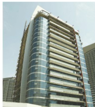
DUBAI-Oasis 1 & 2 Tower Investors - Dubai Sports City
